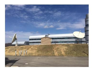
In Sept. 2022, NOAA replaced the existing omni-directional backup pilot uplink antenna installed on the roof of CBU with two 3.8m parabolic antennas similar to the primary pilot uplink antennas at WCDAS.
